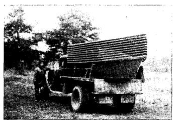
FIGURE 68.—Engineer 1½-ton dump truck with normal load of 10 assault boats.
