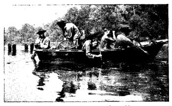
FIGURE 45 .-- Assault boat used to carry anchor cable across stream.
